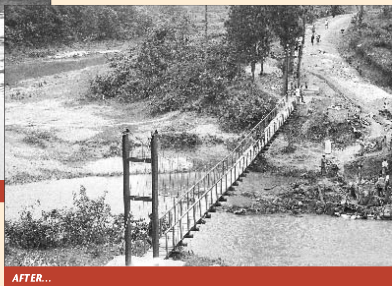
First suspended footbridge in Rwanda, constructed by KIST students and visiting German students and funded by the German embassy
