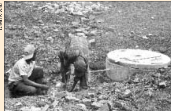
David Mwarira A digester under construction
