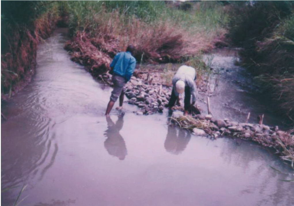
Photo 4.1 Intake of Kalanzi Traditional Irrigation Scheme
